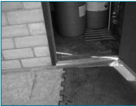
Before worksite modification – barrels have to be moved by hand
