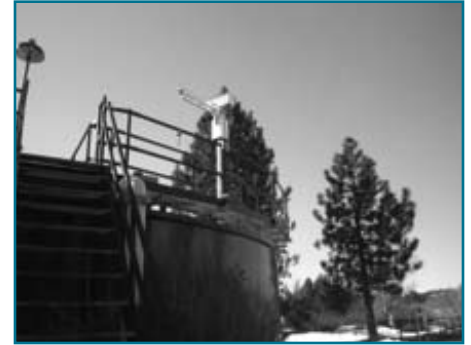
After worksite modification – equipment hauled by jib crane
