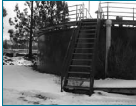
Before worksite modification – equipment carried up stairs by hand
